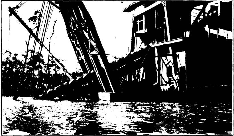
Fig. 1. Digging ladder of the Malaguit dredge on Malaguit River, Camarines, showing the close-connected, 5-cubic foot buckets filled to capacity.
